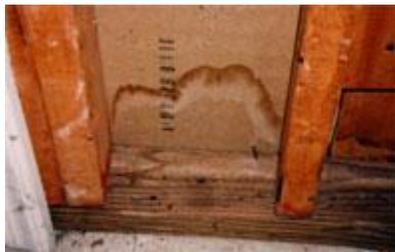
Water stain on a basement wall -- locate and fix the source of the water promptly. [Click on the image for a larger version.](#)
