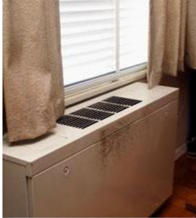
Mold growing on the surface of a unit ventilator. Click on the image for a larger version.
